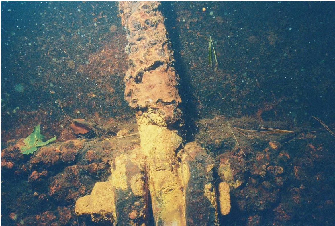
PHOTO #5 SHOWING CONNECTION OF STEM TO GATE, NOTE THROUGH FASTENER
