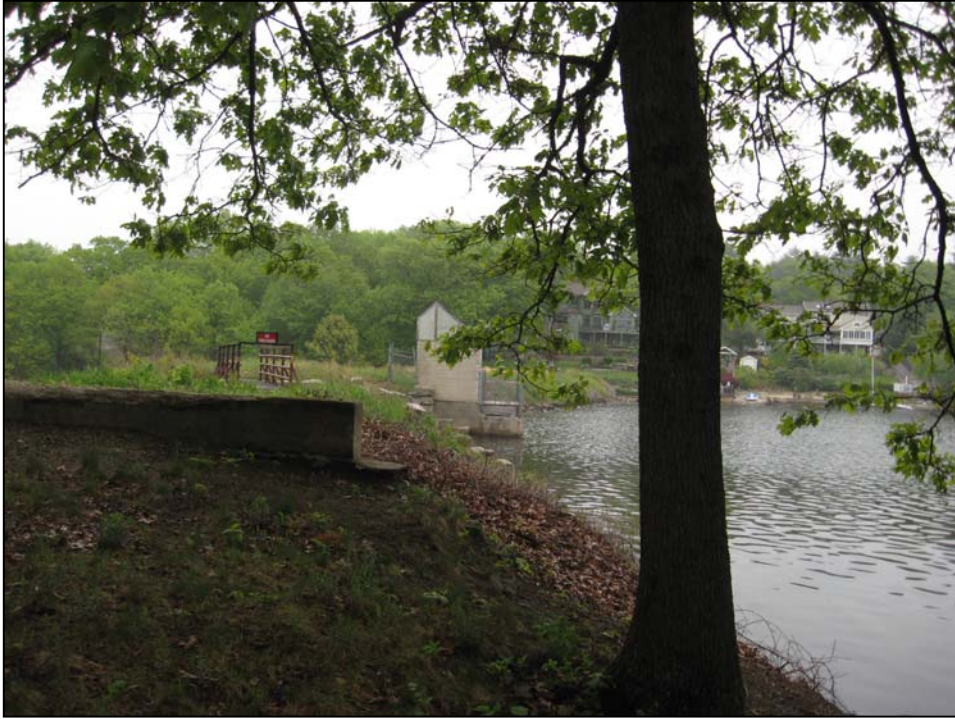
Photo No. 1: Overview of upstream slope from the left abutment.
