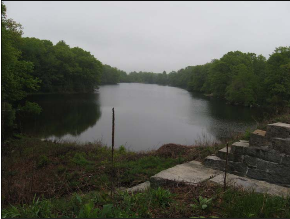
Photo No. 25: Overview of the downstream area as viewed from the primary spillway.
