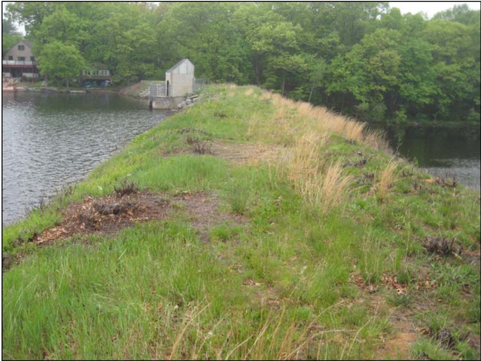
Photo No. 10: Overview of crest from the right abutment.
