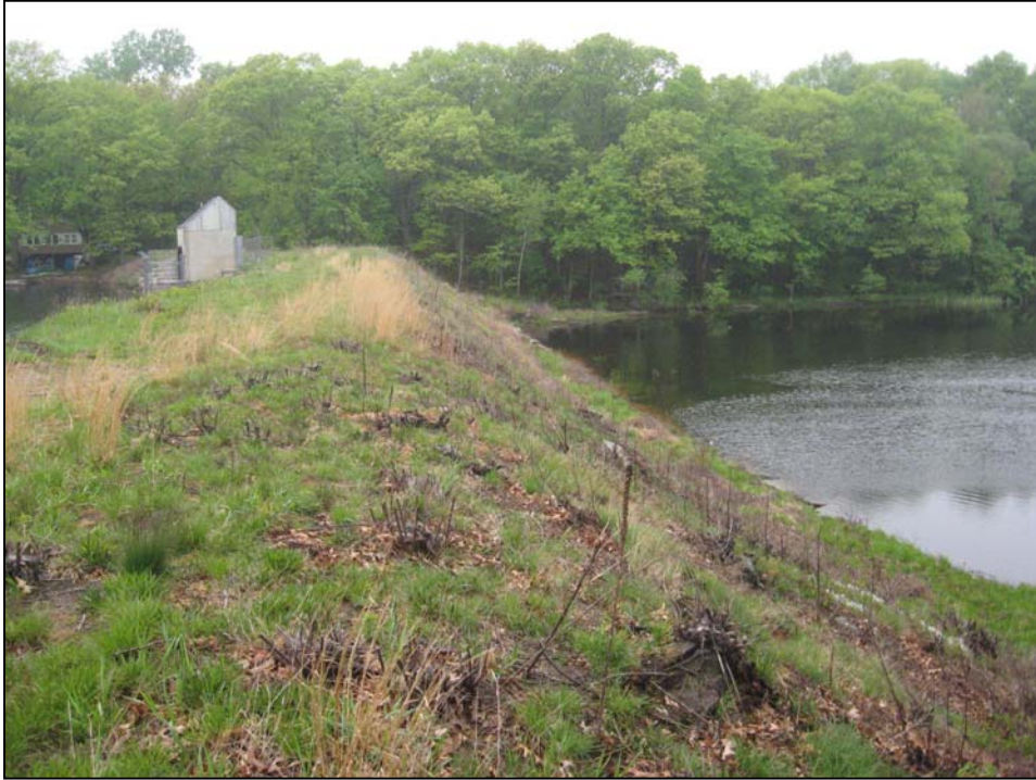
Photo No. 15: Overview of downstream slope from the right abutment.
