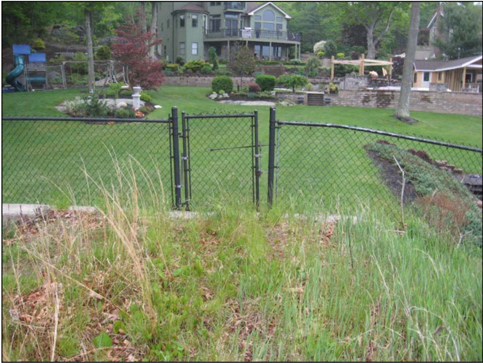
Photo No. 9: The right abutment looking right.
