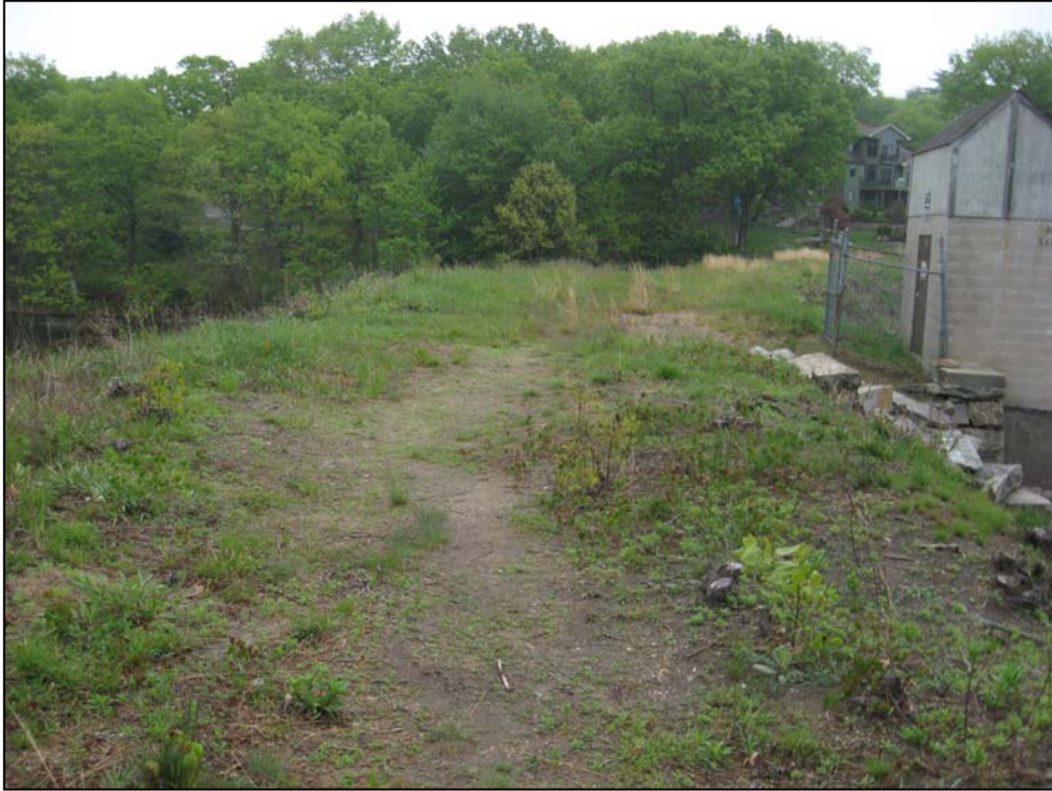
Photo No. 7: Overview of crest from the primary spillway looking right.
