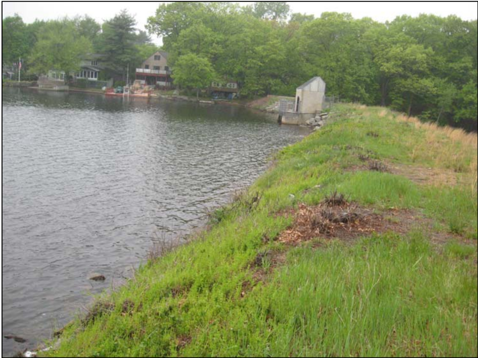
Photo No. 4: Overview of upstream slope from the right abutment.
