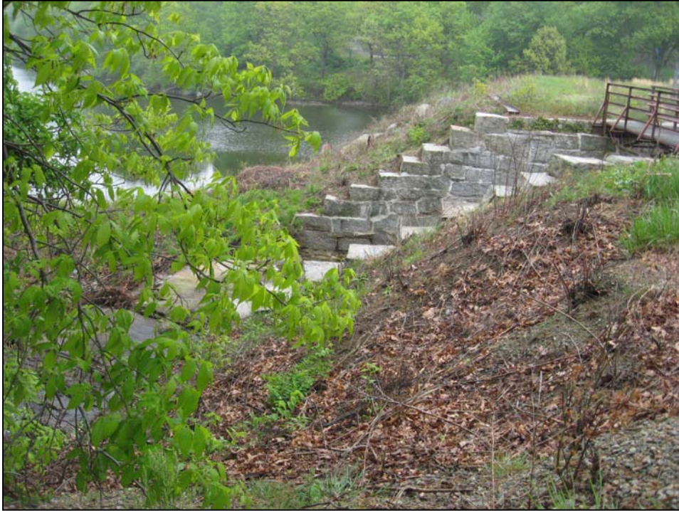
Photo No. 11: Overview of downstream slope from the left abutment.
