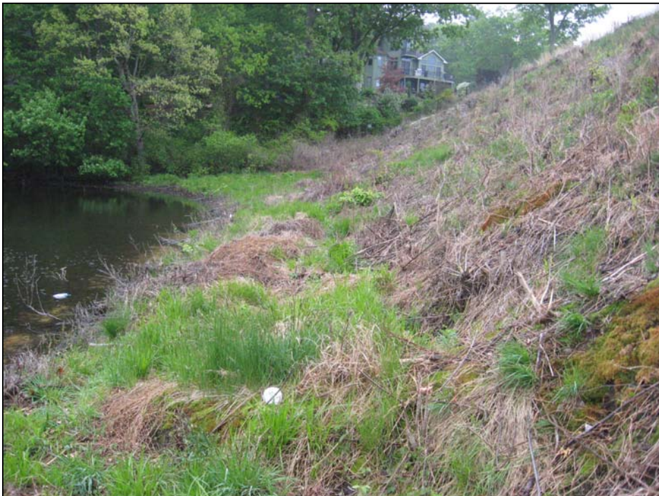
Photo No. 16: Downstream slope as viewed from Station 2+50 looking right.
