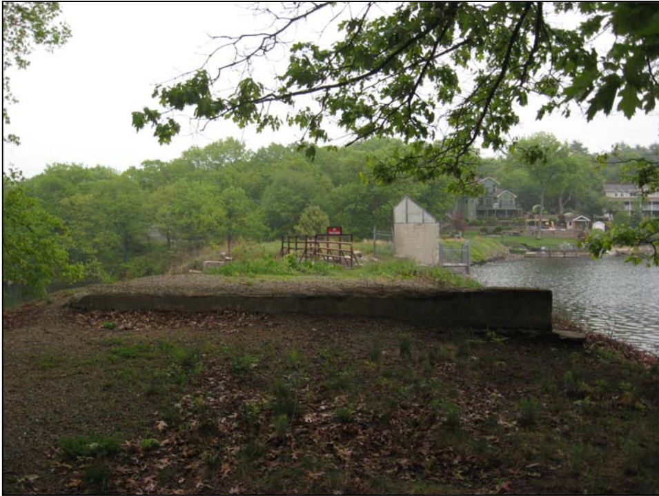
Photo No. 5: Overview of crest from the left abutment.
