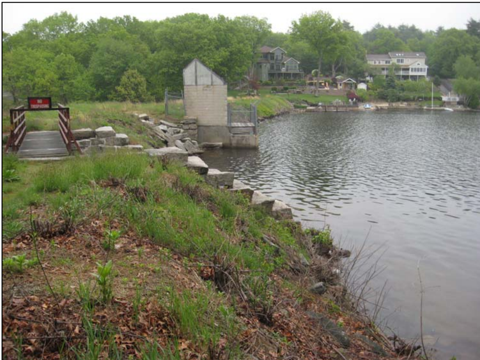
Photo No. 2: Overview of the upstream slope in the area of the primary spillway looking right.
