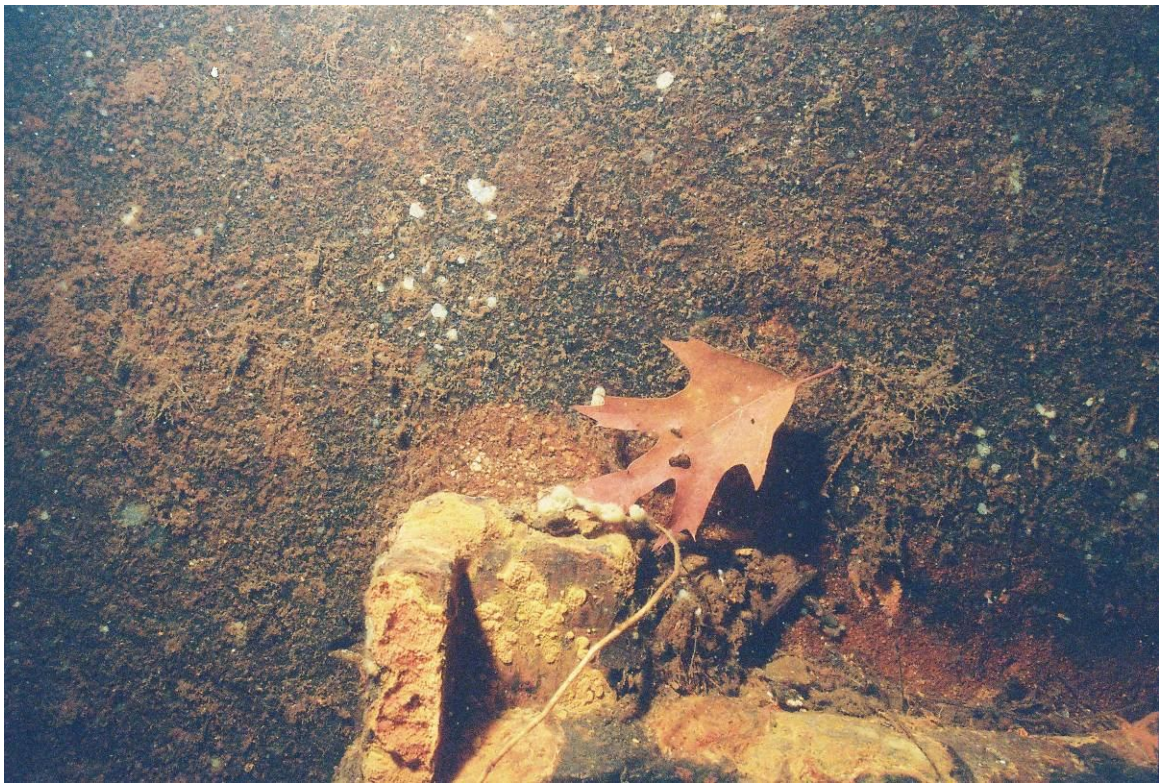
PHOTO #6 SHOWING TOP OF GATE GUIDE, CAMERA FACING FLOOR
