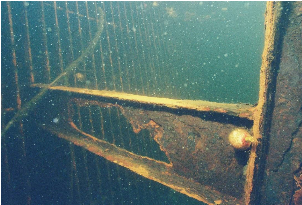
PHOTO #4 SHOWING HORIZONTAL BRACE WITH PERFORATED WEB SECTION
