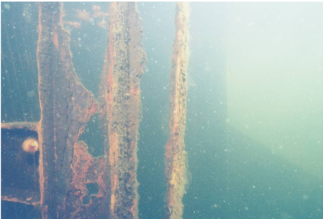
PHOTO #3, SHOWING VERTICAL I BEAMS WITH PERFORATED WEB SECTION
