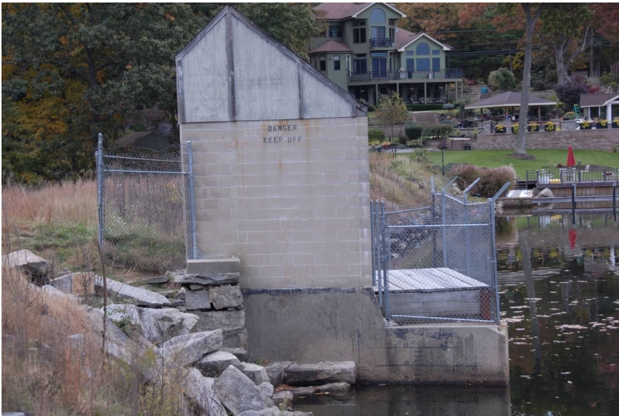
Photograph No. 1, gate house
