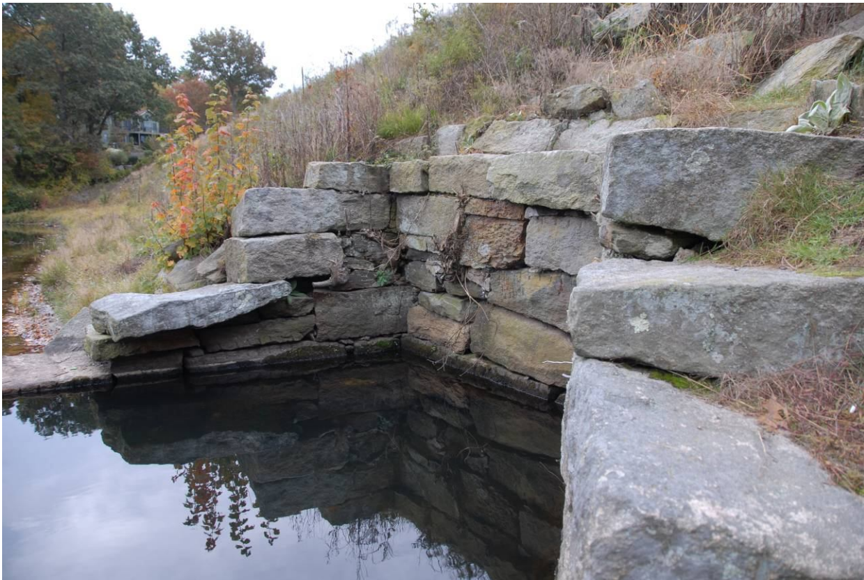
PHOTO #8 SHOWING DISCHARGE STRUCTURE AT END OF 36 INCH PIPE DOWNSTREAM
